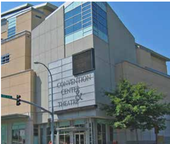
Meydenbauer Center helps form the eastern portal of the Eastside Center District
